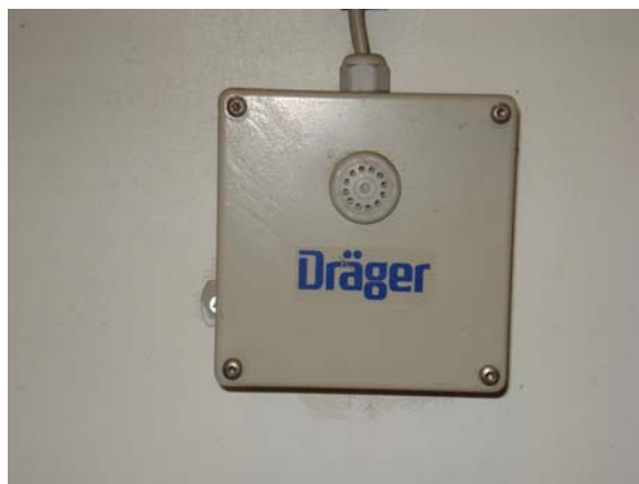
LPG/propan-detektor.
