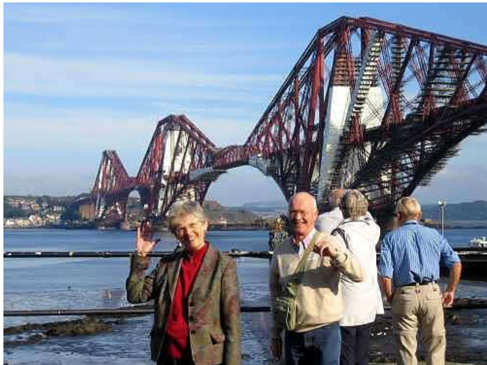
Firth of Forth bridge
