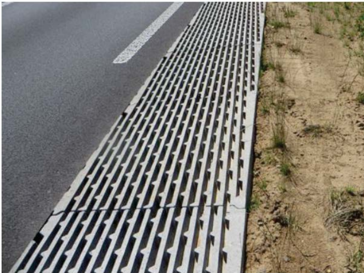
Figure 1. Whisstone diffracting elements variant 1 (section 1)
