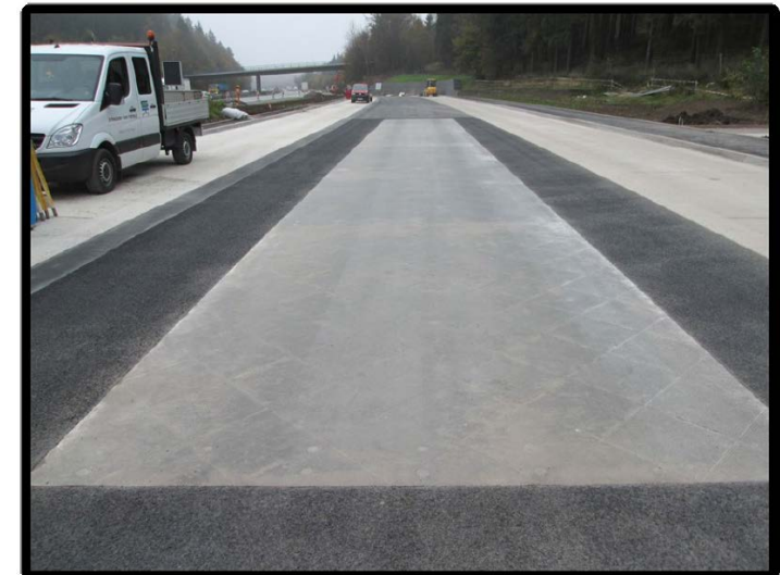
Figure 7 –test track of low noise surface in UHPC
