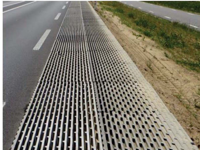
Figure 2. Whisstone diffracting elements variant 2 (section 2)
