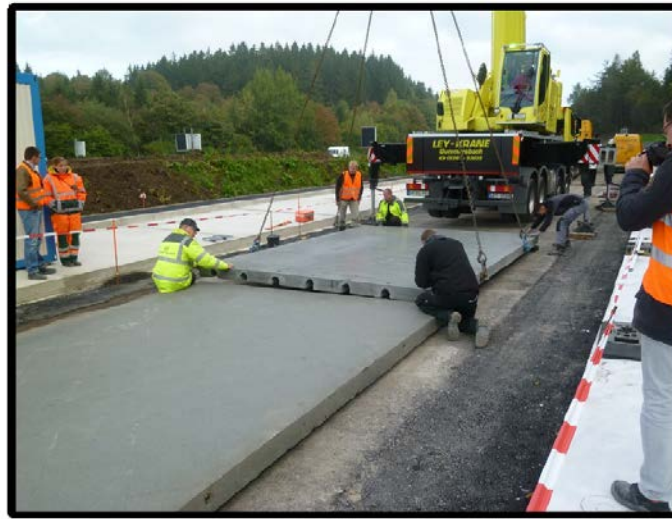
Figure 6 – laying of low noise surface in UHPC precast elements
